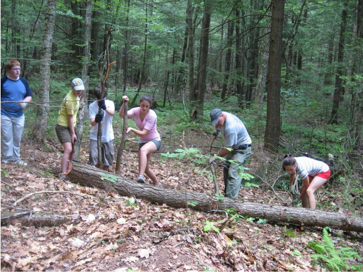
Tilton Farm trail construction crew, June 2010
